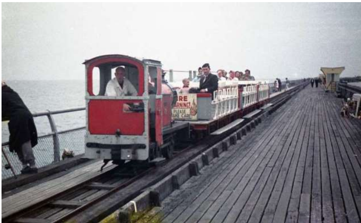
The train is seen returning from the Pier Head back to the shore end. Note the wooden troughing alongside the track used to guide the 1936 pneumatic tyred car. The fisherman leaning over the Pier railings seems undisturbed by the train's passing.
