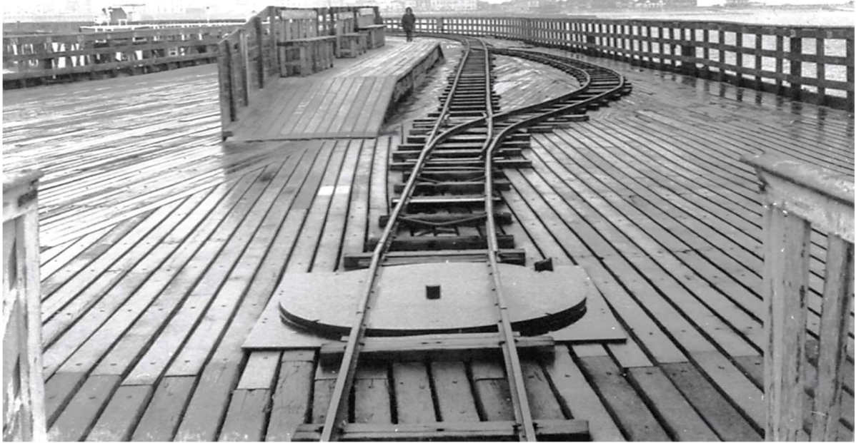
A view of the Pier head station looking back towards Walton-on-the-Naze on a damp, dismal day. The small turn plate in the headshunt can be clearly seen. Whether it was ever used to turn the locomotive is not known. The curve in the Pier is noticeable in this view.
