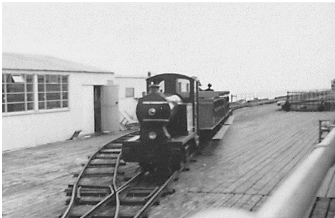
Taken in 1949 a year after opening, this is the earliest known photograph of the railway. Baguley 0-4-0PM 3024, probably little changed since arriving at Allhallows-on-Sea in 1939, is seen at the shore end station. This was then a simple affair, set at an angle across the Pier, with a run-round loop but no platform. The track was directly on the Pier decking.
